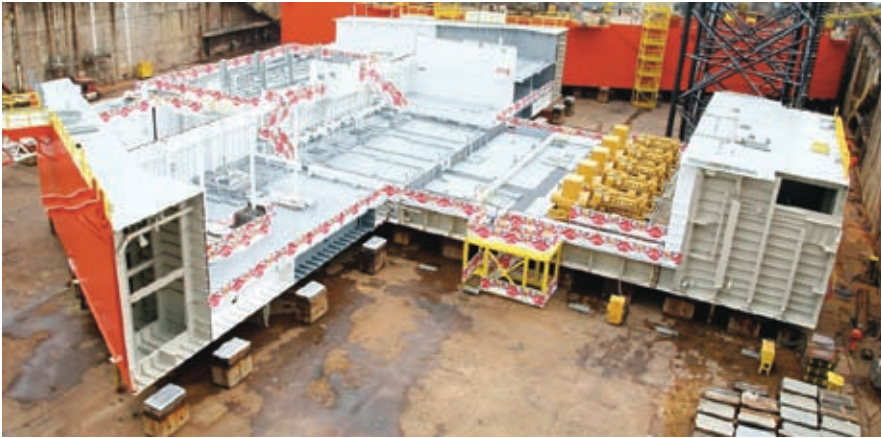
On-track progress for West Juno's hull at Keppel FELS
