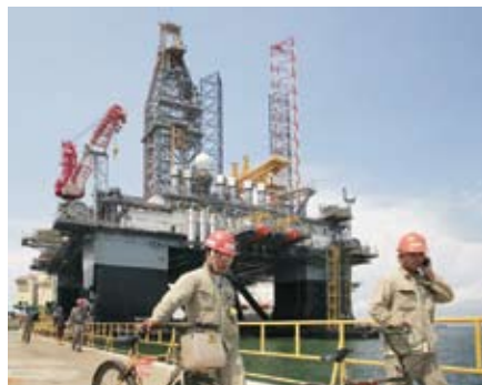
Keppel FELS is currently constructing another six similar semis for ENSCO
