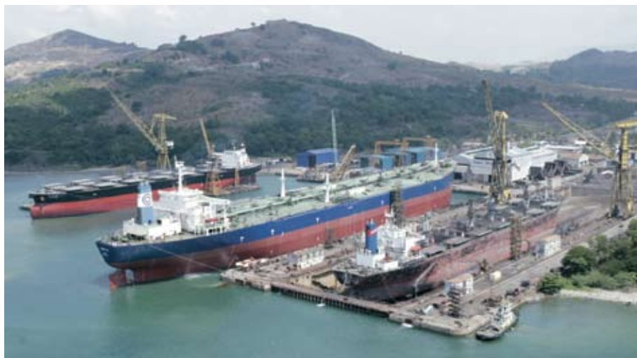
The extension of the lifting capacity radius will mean double banked vessels have the full service of the crane
