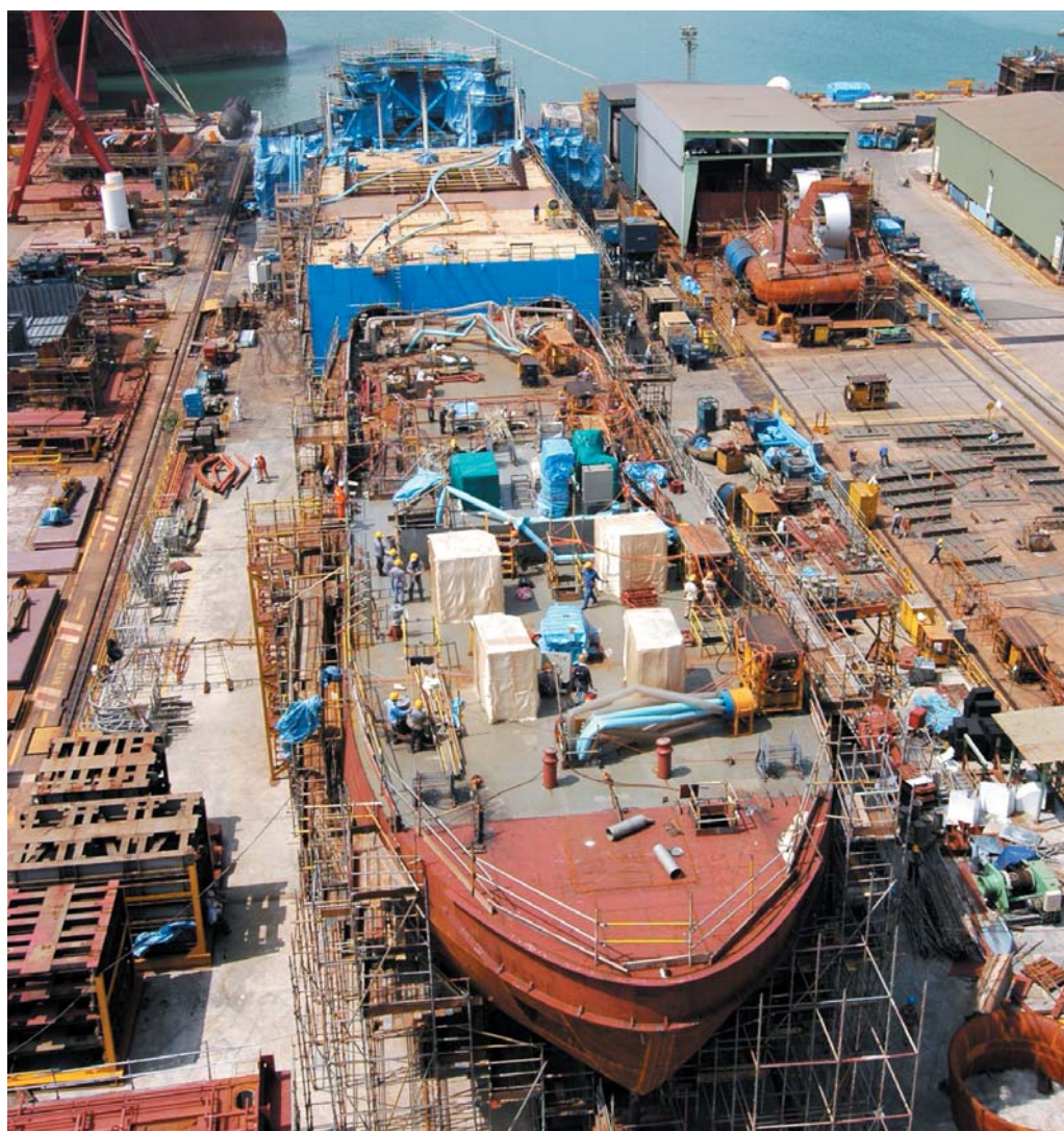
An icebreaker is shown here under construction at Keppel Singmarine's Benoi yard
