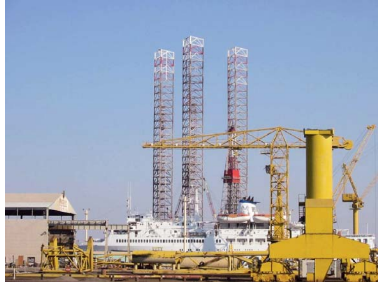
The Perronegro rig towers in the background while the Car carrier, AJMAN CITY, is engaged in the bustle of the yard
