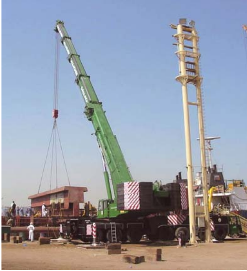
Lifting and installation of the separation wall for the HAM 602
