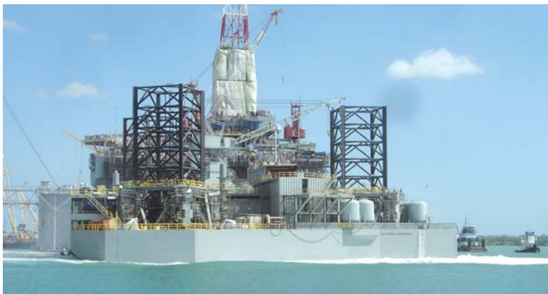
Offshore Courageous takes to the water at Keppel AmFELS
