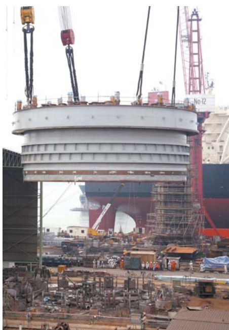
Excellent execution during the lifting and installation of the upper turret for P-53
