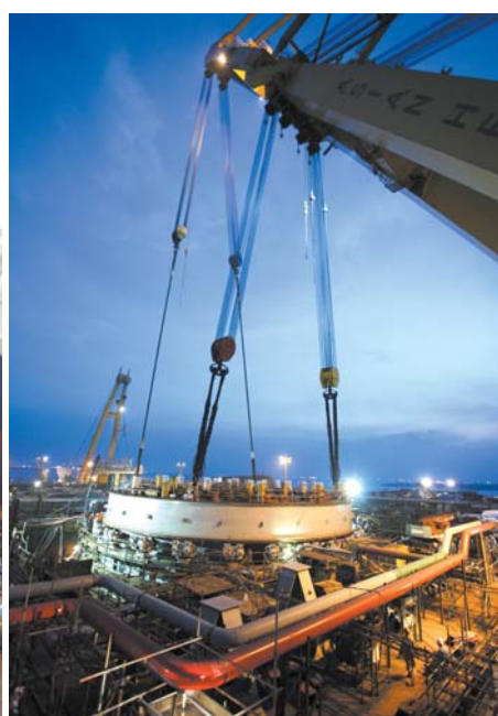
Excellent execution during the lifting and installation of the upper turret for P-53
