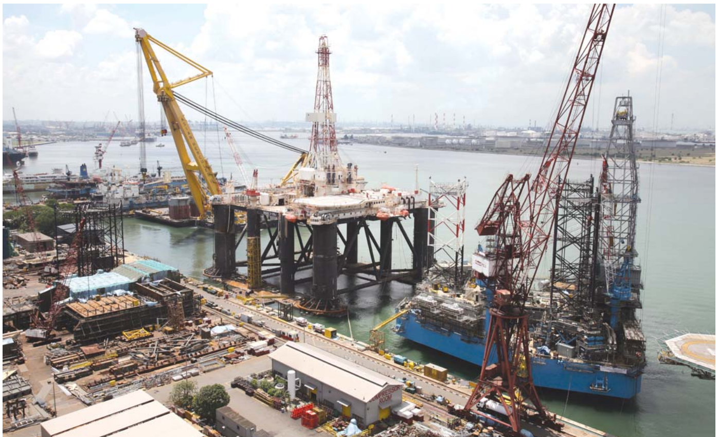
Keppel FELS and Keppel Verolme will each undertake the upgrading of a Sedco 700-series semisubmersible drilling rig for Transocean. Shown above (left) is the semisubmersible that Keppel FELS is upgrading
